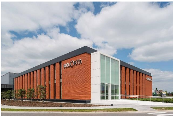
Figure 11: BelOrta Building (Architectenvenootschap ar-te bcvba, 2015a)
