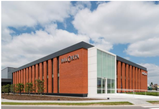
Case study 1: BelOrta building of ar-te in Belgium
