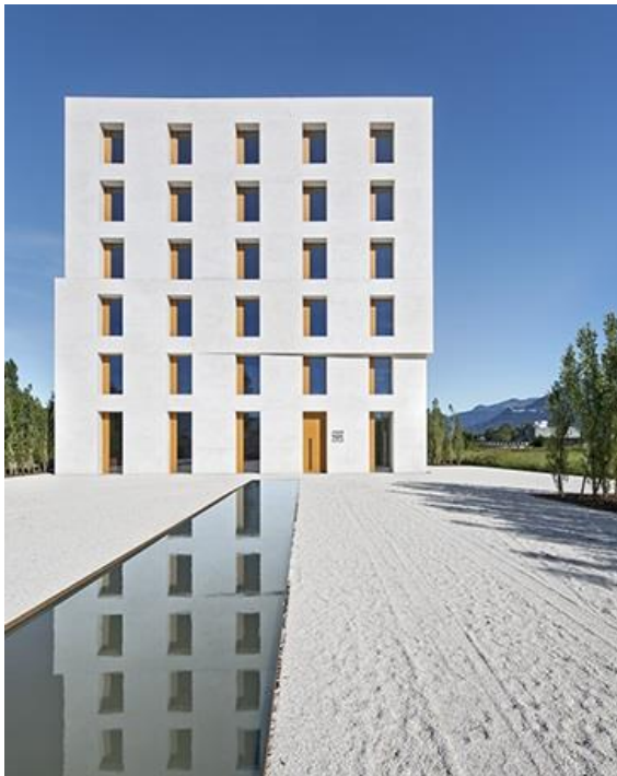
Figure 13: BE2226 building (Source: www.baumschlager-eberle.com/projekte/projektetails/project/buerogebaeude.html )
