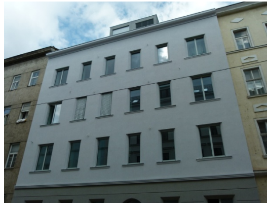
Object Eberlgasse, 1020 Vienna - First modernization of a historic building to passive house standard - water/water heat pump - air ventilation system
