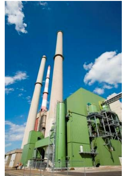
Biomass cogeneration plant: Simmering/Vienna.
